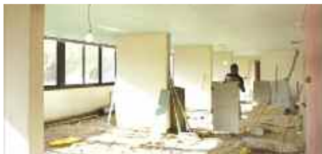
Rehabilitation of the Cafeteria at the loF first floor
